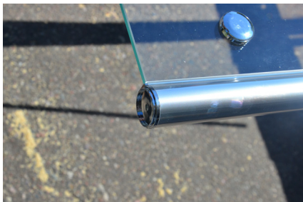
Install base for tie bar receptor.
