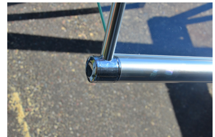
Add decorative cap onto tie bar receptor.
