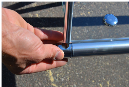
Install tie bar receptor and tie bar.
